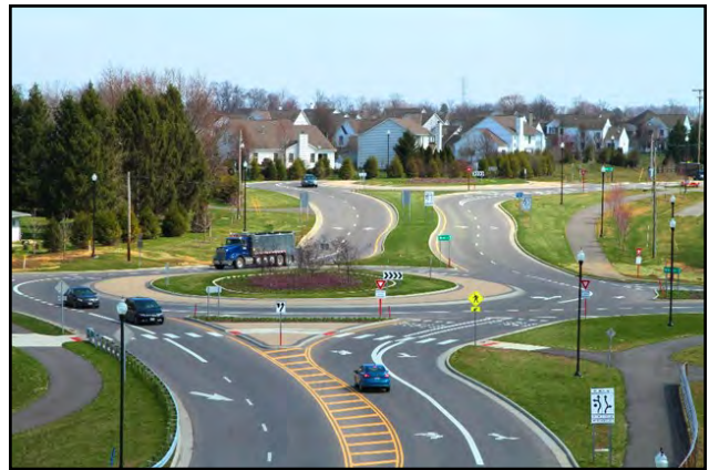
Modern, low-speed roundabout; South Section Line Road and Riverside Drive, Concord Township. Pedestrian crosswalks are behind the pause line for traffic. Safe design speed is 11 miles per hour.
