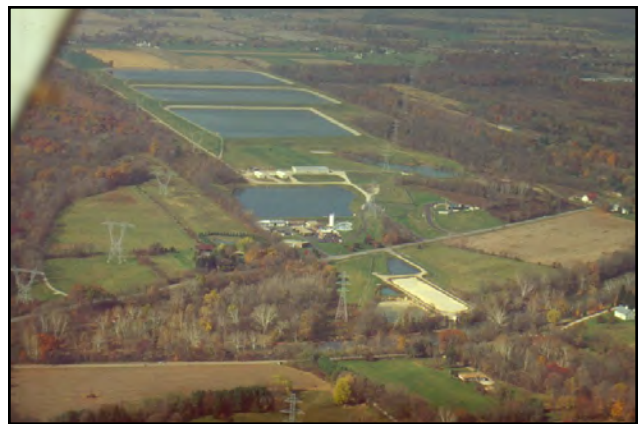
Del-Co Water Headquarters on S.R. 315, Liberty Township
